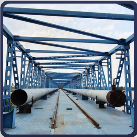
DAM WATER PIPELINE BRIDGE
